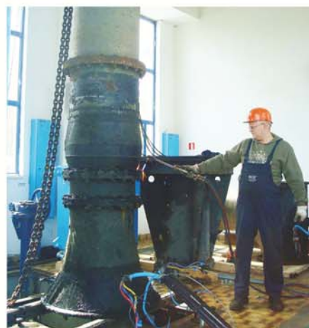
Remont pumpe 3500 l/s
